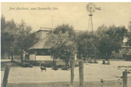
Port Maitland, near Dunnville, Ont.
